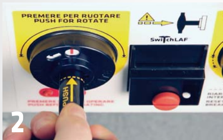
drawer in "disconnected" position
