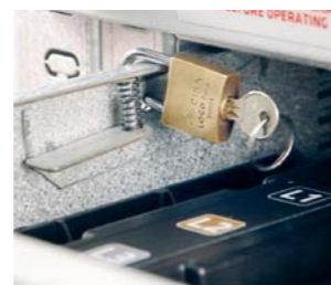
Safety: • safety of "withdrawn drawer". • safety of "not connected drawer".
