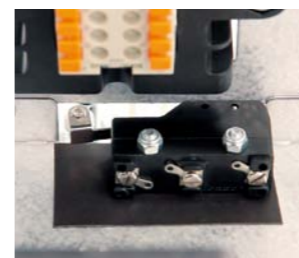
Position switches: • position switch "disconnected drawer". • position switch "withdrawn drawer".
